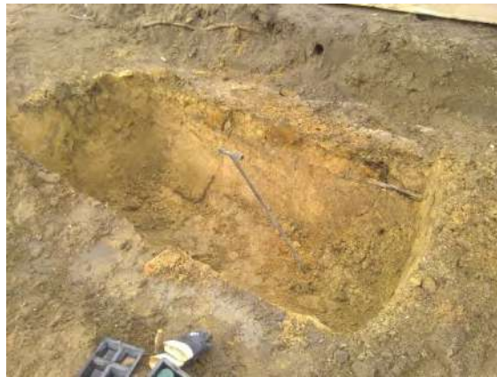
Foto 12 controle na tanksanering dmv olie-watertesten
